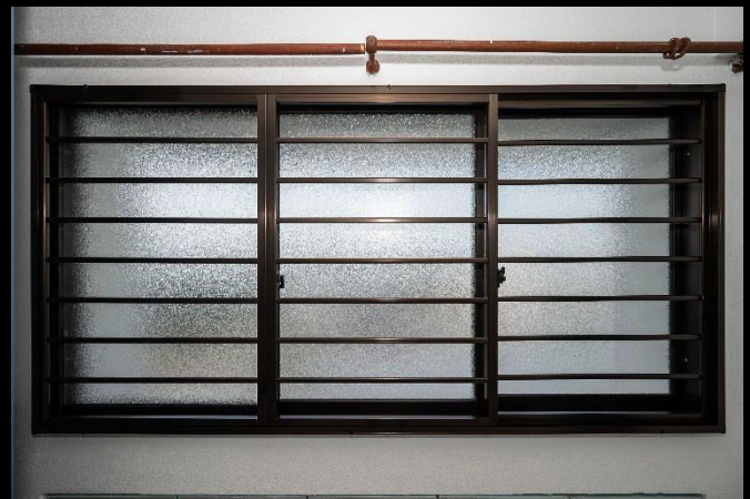
Sliding Window with Grilles Bronze Frame with Orange Skin Glass
