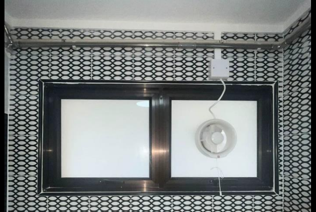
Top Hung Window with Ventilation Fan (Bronze Frame with Frosted Laminated Glass)
