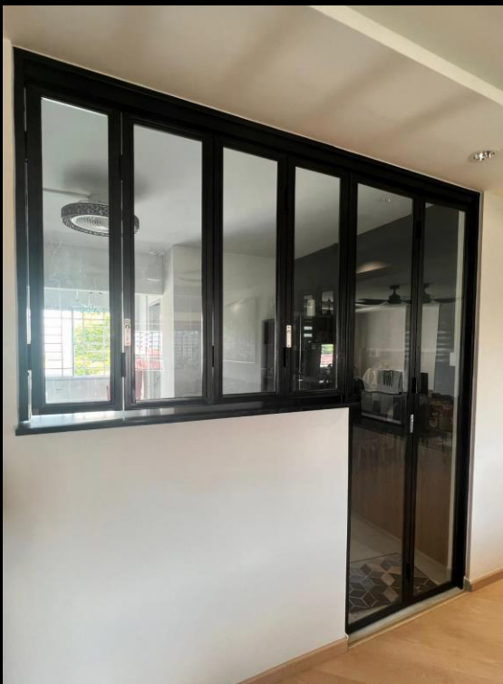
Mild steel top hung bifold glass door and mild steel bifold window
