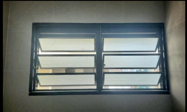
Louvre Window (Bronze Frame with Wired Glass)
