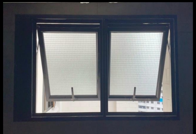
Top Hung Window (Bronze Frame with Wired Glass)
