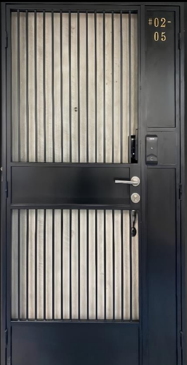
Gate design with uneven flushed side plate
