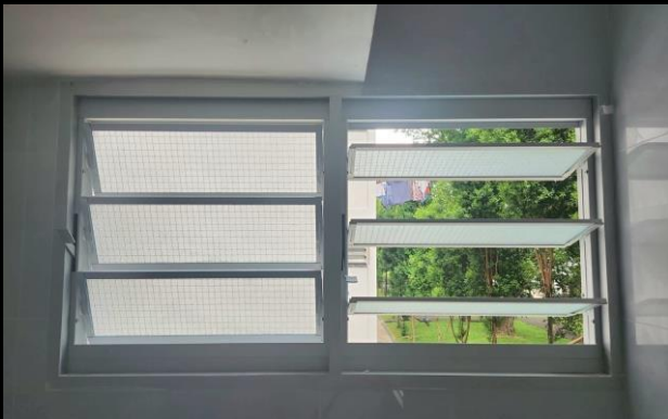
Louvre Window (Silver Frame with Wired Glass)
