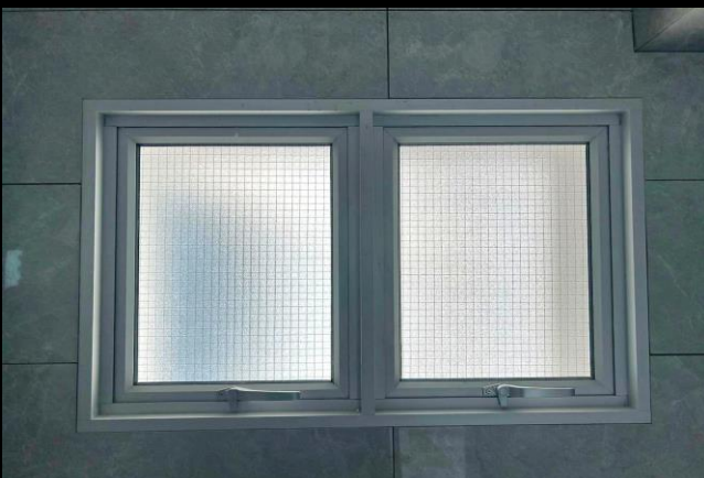
Top Hung Window (Silver Frame with Wired Glass)
