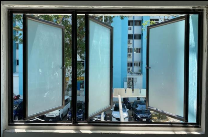
Casement Window Bronze Frame with Frosted Glass
