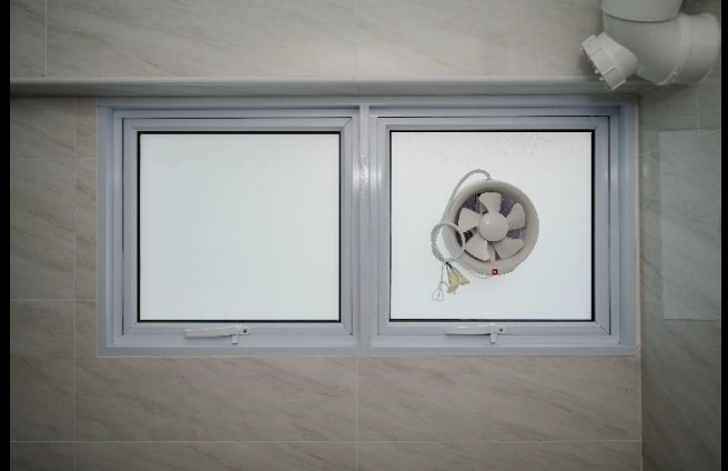
Top Hung Window with ventilation fan (Frosted laminate glass with white frame)
